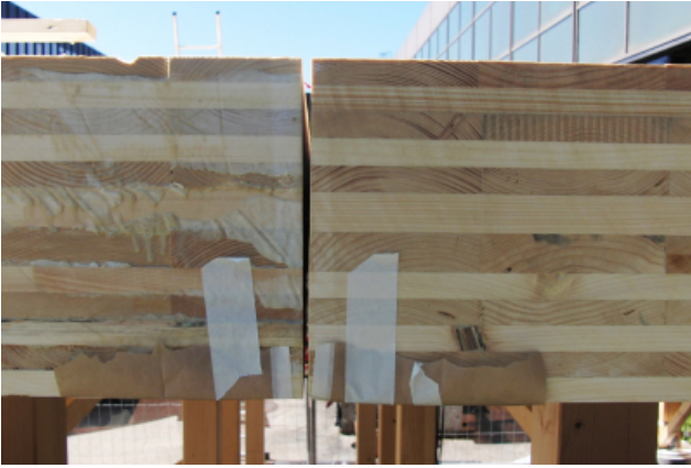
Joint ready for bonding
