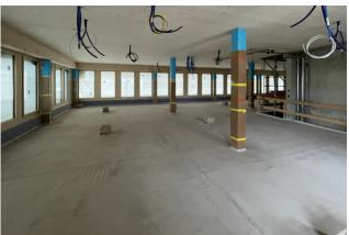
The new Raiffeisenbank Wasserschloss building in Gebenstorf, designed by Merlo Architekten AG, is based on the TS3 skeleton construction method: Columns and wide-span, point-supported cross-laminated timber panels form the load-bearing structure, so that surrounding ribbon windows create an open and bright ambience. The wide-span load-bearing structure enables a flexible room layout for the counter hall and the office space above, which is spread over the other three floors.
