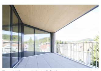
Thermal bridges made simple. CLT ceiling simply runs through from the apartment to the loggia.
