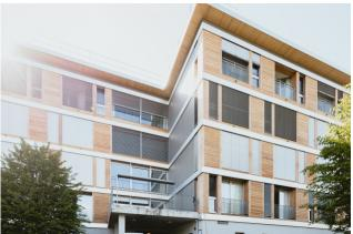
The retirement and care center in Esslingen needed additional space. Thanks to the innovative TS3 technology, the existing load-bearing structure could be taken over and the building extended by 2 storeys. The short construction time, use of regional timber and flexible room design thanks to TS3 technology make the building a showcase project for sustainable construction
