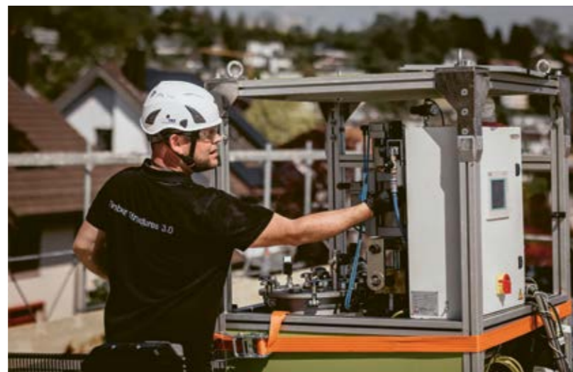
Potting TS3 connection on site with casting equipment
