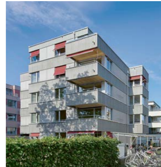
Apartment building Wehntalerstrasse, Zürich
