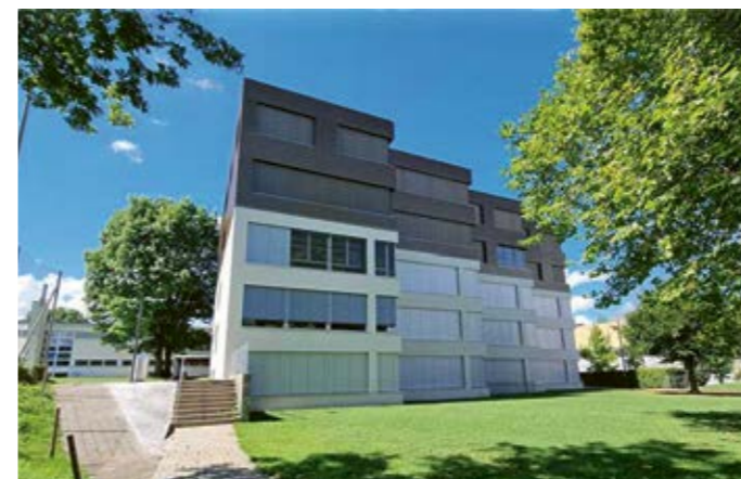
School building Feld 1, Richterswil
